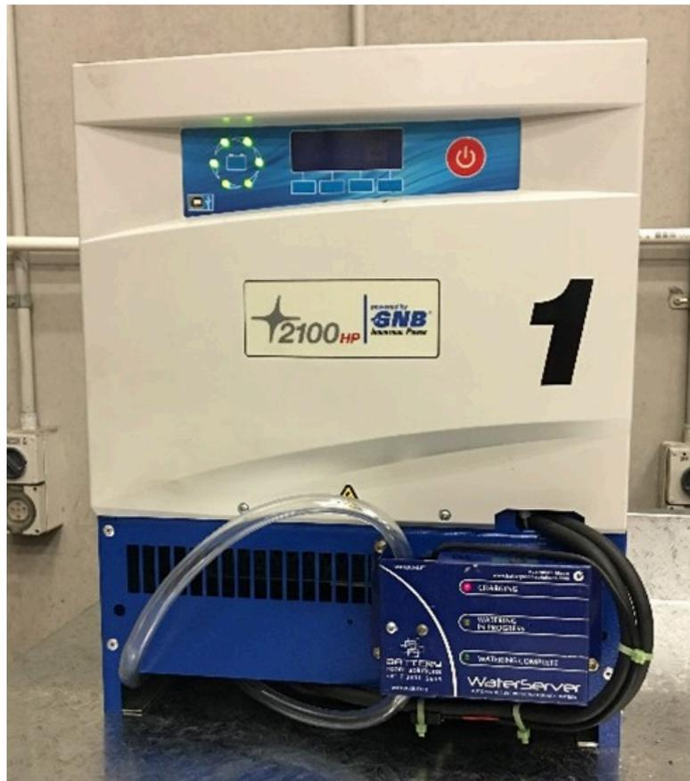
Figure 4. WaterGenius mounted to front face of Battery Charger
